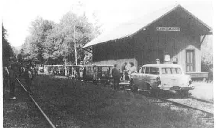
A lineup of track cars (and one HyRail car) are shown at Fleischmanns, New York, during the NARCOA fall meet on the Delaware & Ulster Railroad.
