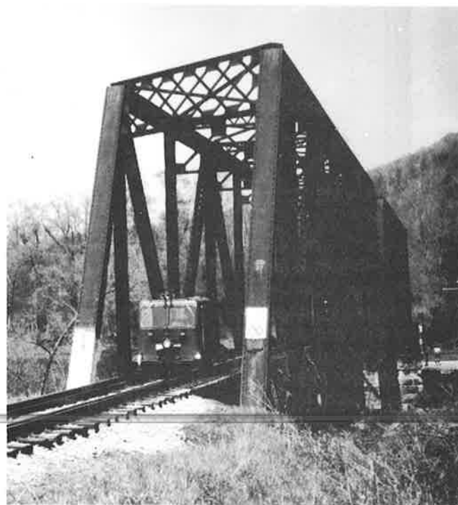
Don Harbaugh's CN MT14 on a truss bridge crossing Oil Creek on the OC&TRR May 18, 1996.
