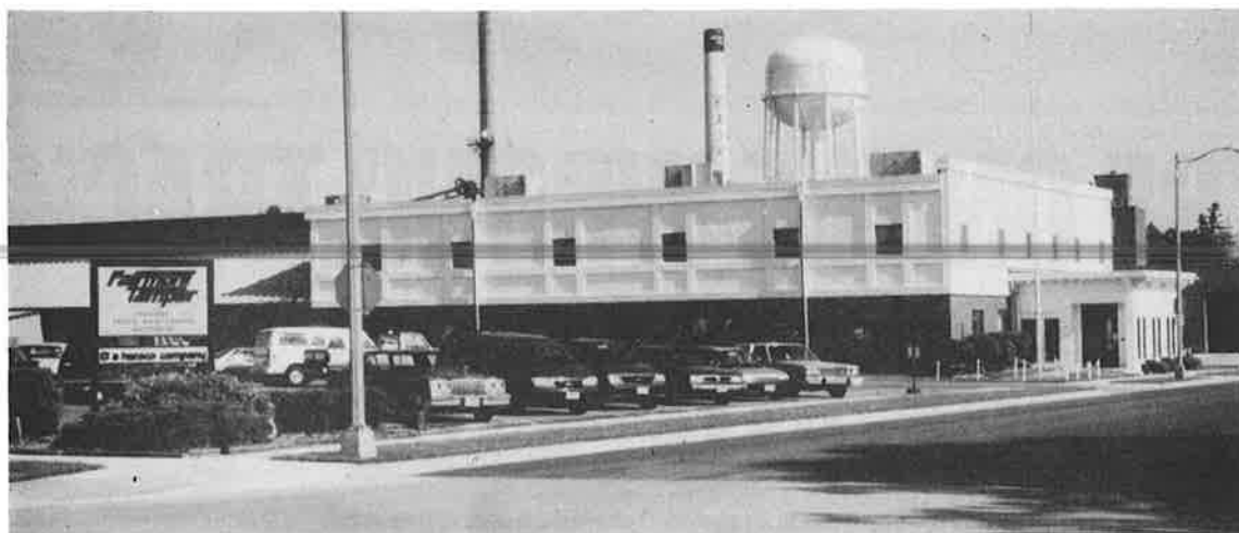
At left, the Fairmont Tamper plant in Fairmont, Minnesota. The original two-story brick and stucco building is on the right while a modern prefab metal addition shows to the left (rear).
