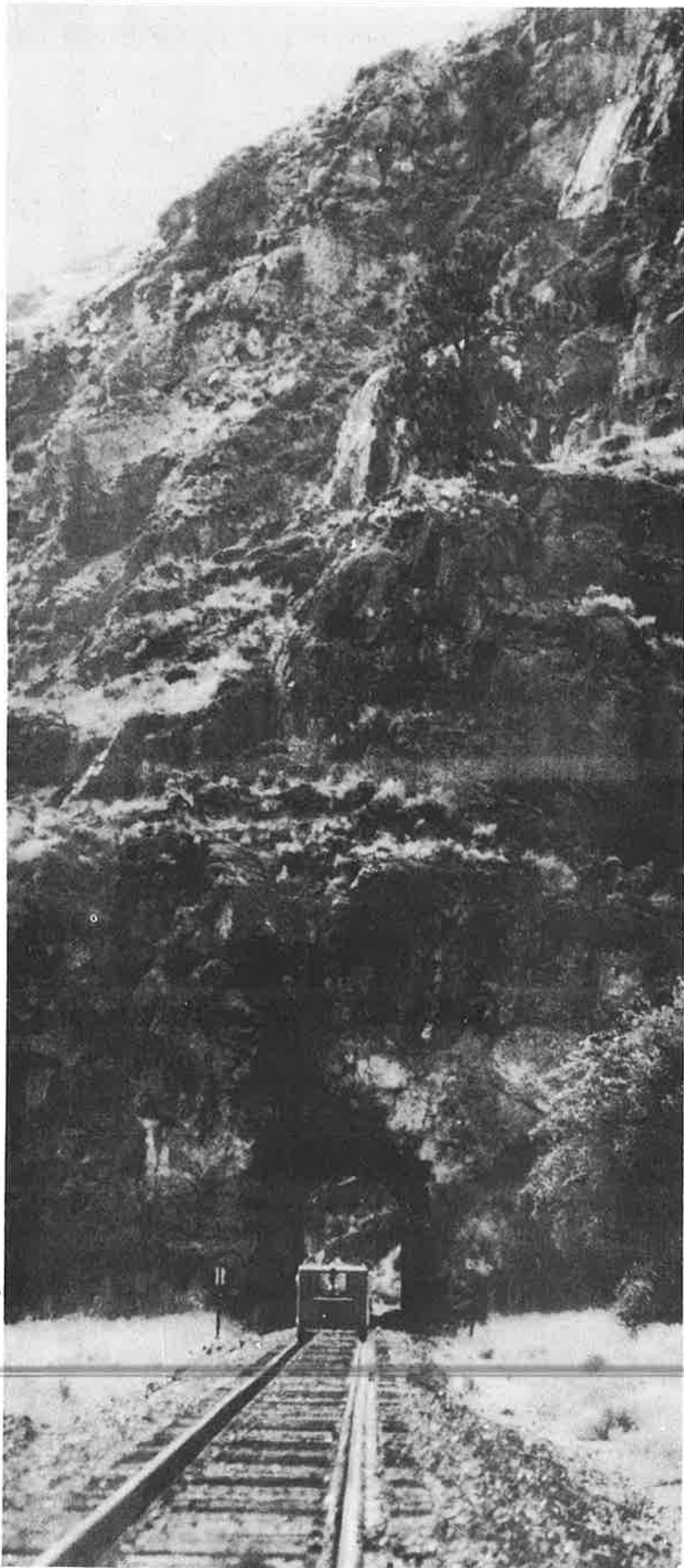
Cascade & Columbia River Railroad's only tunnel, MP 35.2. Photo by B. Douglas Jensen
