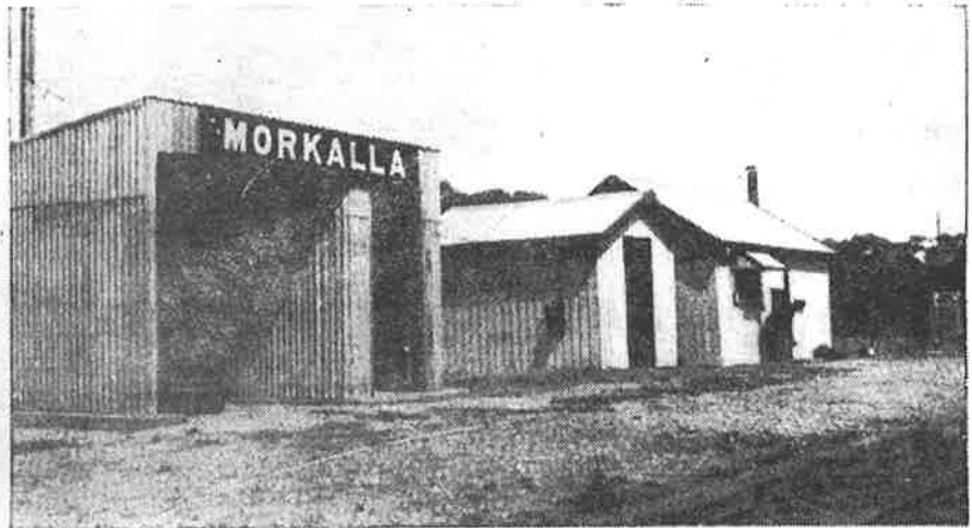
Morkalla station, showing rest huts for train crews.
