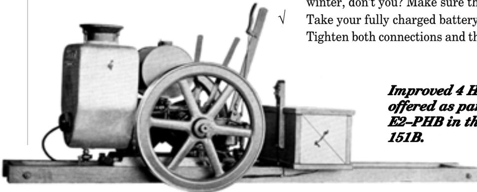
**Improved 4 H.P. PHB Motor Car Engine, offered as part of Motor Car Outfit E2-PHB in the 1936 Fairmont Bulletin 151B.**
