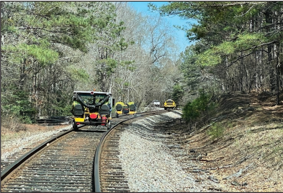
Rolling along through sweeping curves on beautifully maintained track
